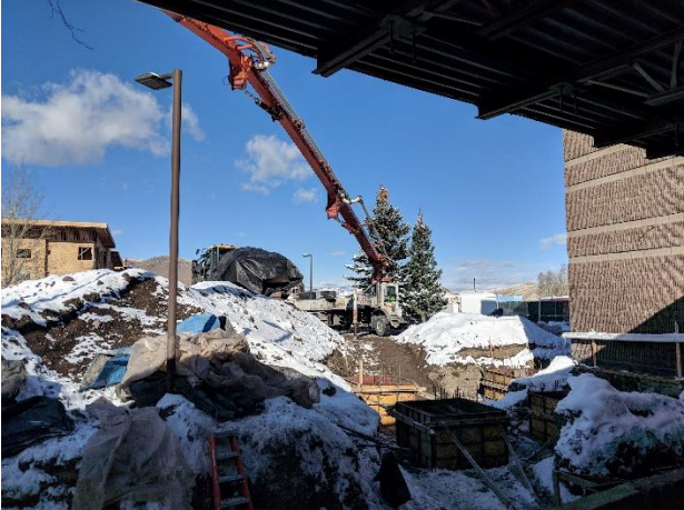
Concrete Foundation Pours: November 8, 2018
