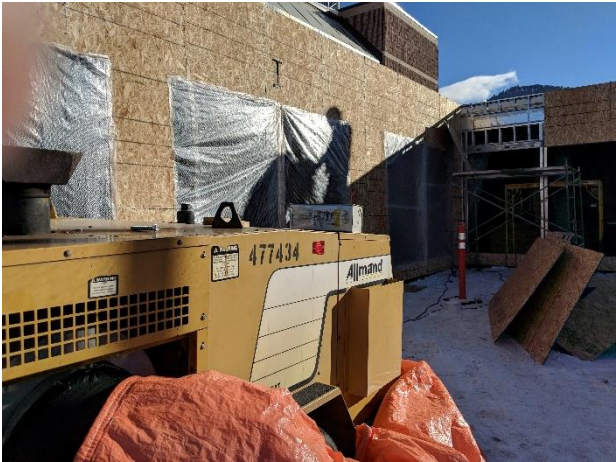
Exterior Walls Going Up: January 11, 2019
